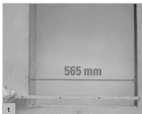
1 Clear installation width required 565mm.
